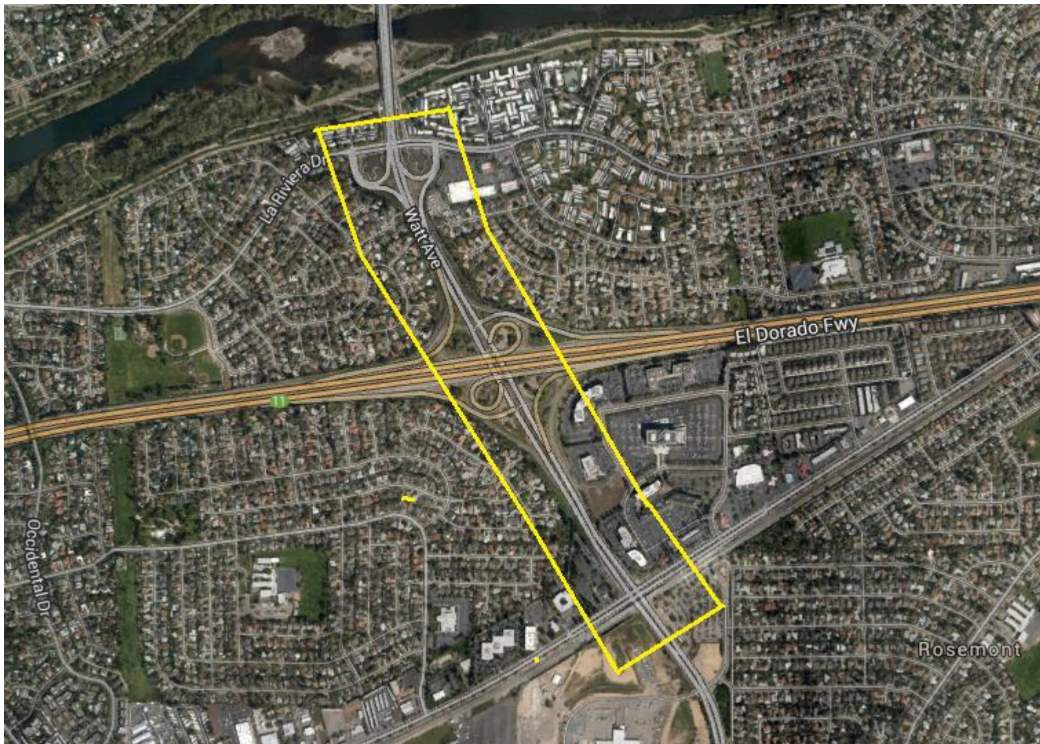
Bus lane added from La Riviera Drive to Folsom Blvd.
